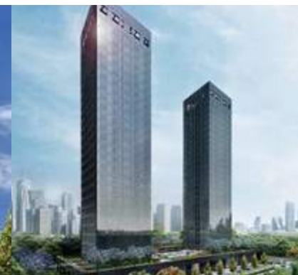
Trump Towers Pune India
